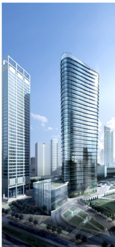
Off-grid/Back-up Large equipment Commercial buildings
